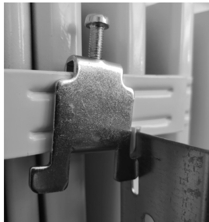
Figure 6 – Locking Clip installed on outside of wall bracket
