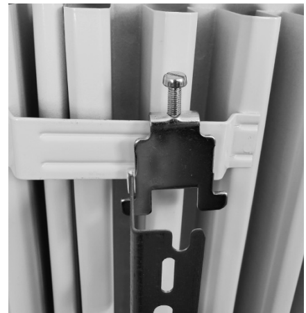
Figure 7 – Locking clip installed towards inside of wall bracket
